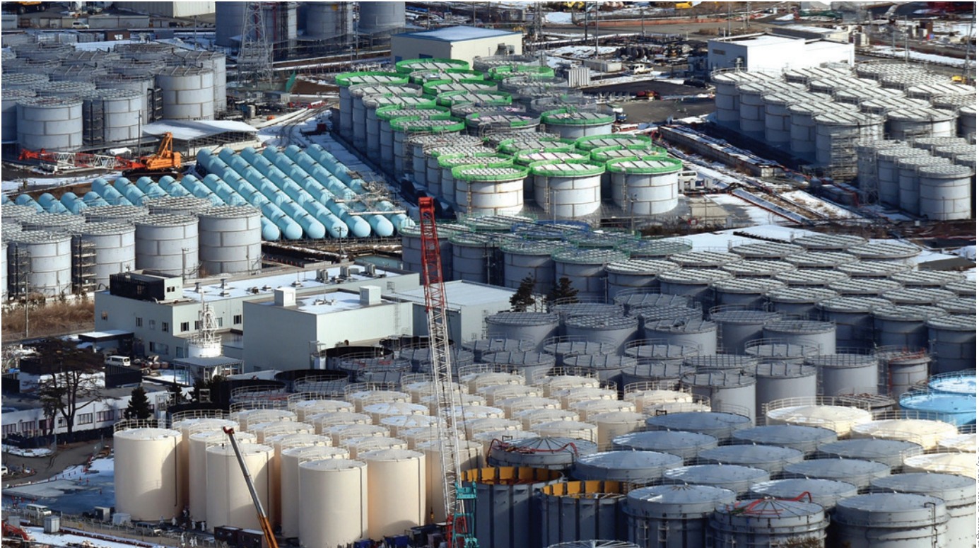
Radioactive cooling water, continuously generated since the Fukushima disaster, is collected in tanks until a long-term storage solution is determined. The NRC's plans for dealing with an American Fukushima could result in a similar buildup of radioactive water.
