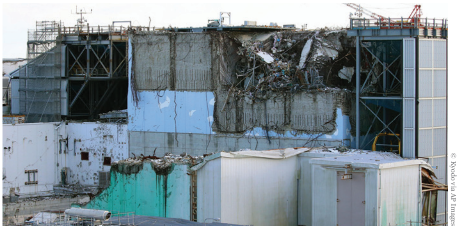
Taken January 25, 2016, nearly five years after the disaster, this photo shows the damage at Fukushima Dai-ichi Nuclear Power Plant's Unit 3 reactor. Unit 3 was the site of a core meltdown and a hydrogen explosion that released radioactivity into the surrounding environment.
